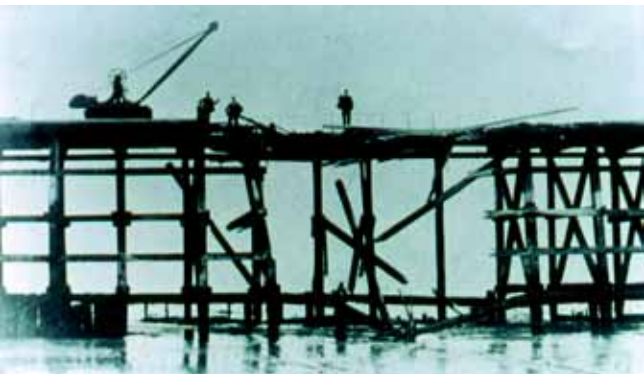
Silloth Pier damaged by shipping
