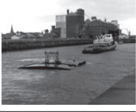
One of the new steel gates being towed into Silloth from Barrow
