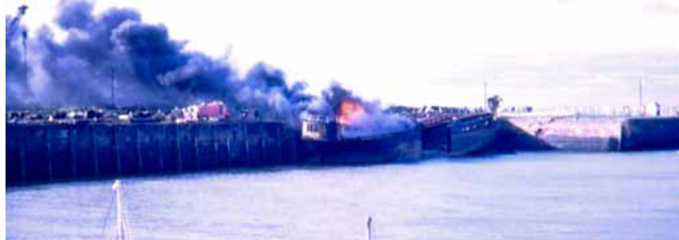
Occasionally, the use of oxy-acetylene torches got out of hand!
