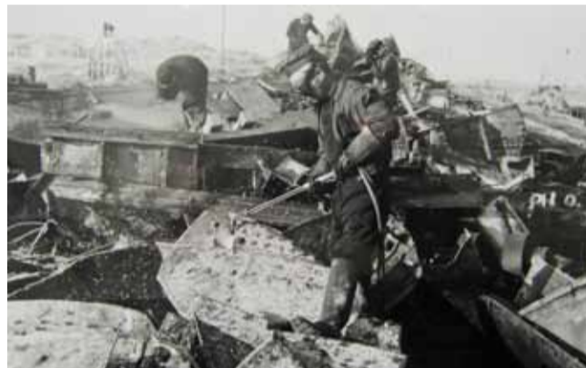
Cutting up the scrap steel with oxy-acetylene torches
