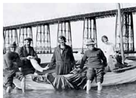
Solway Viaduct, showing the piers, each consisting of 5 interlocked piles
