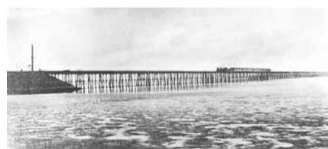
Solway Viaduct, from the English side
