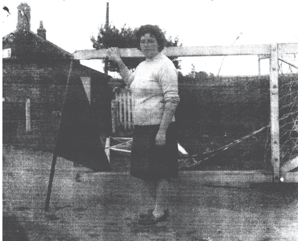
Crossing Keeper Margaret Gass holding the broken section of railway crossing gate
