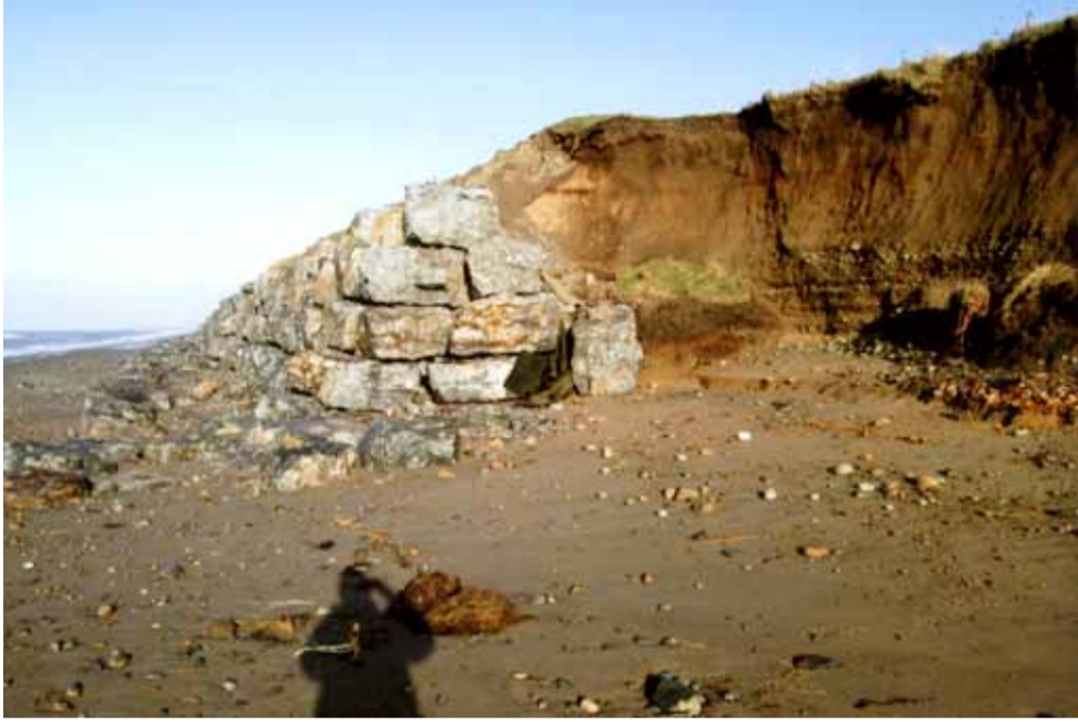
This photograph by Geoff Bland clearly shows the vast amount of damage the tide has caused to the new retaining wall at Beckfoot. An extension of the wall and infilling to protect the coast road is expected to cost £100,000.
