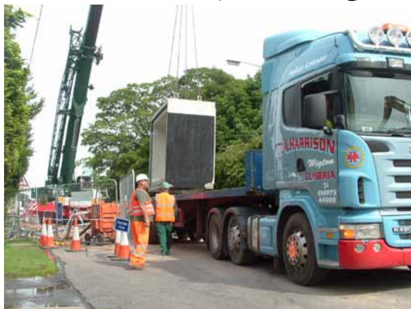
Culvert sections being delivered
