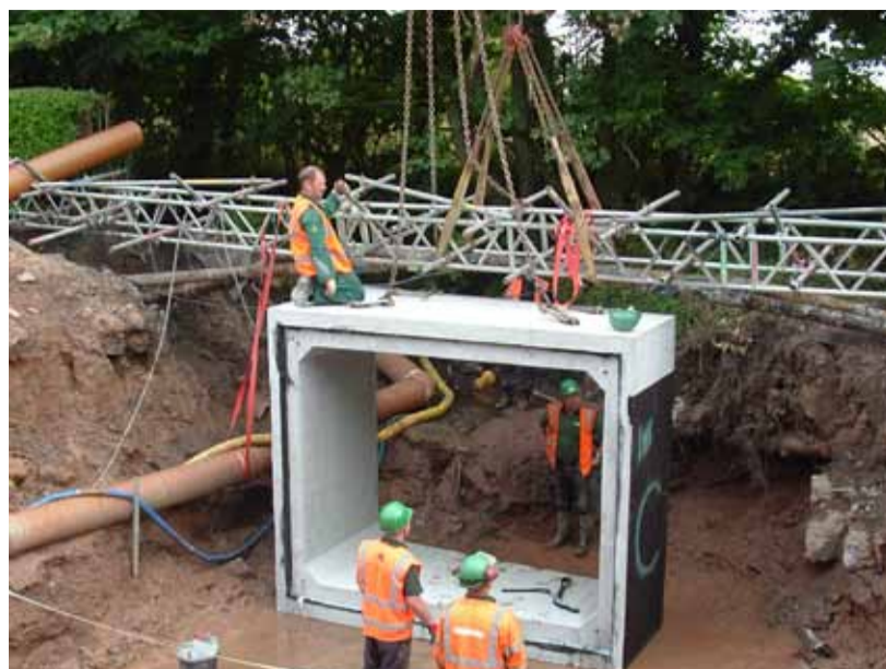
The first section being placed in the gully
